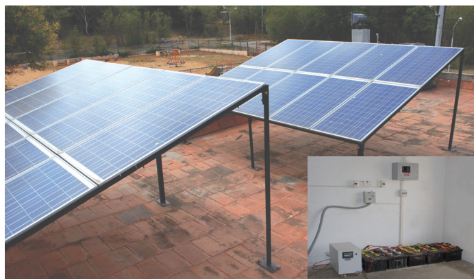
Solar panel and control system (inside view) at CFTRI
